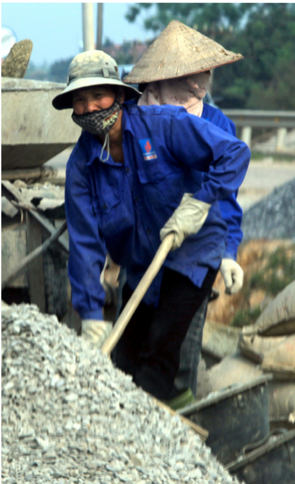
Construction workers at work. © ILO/T. Van Vi
